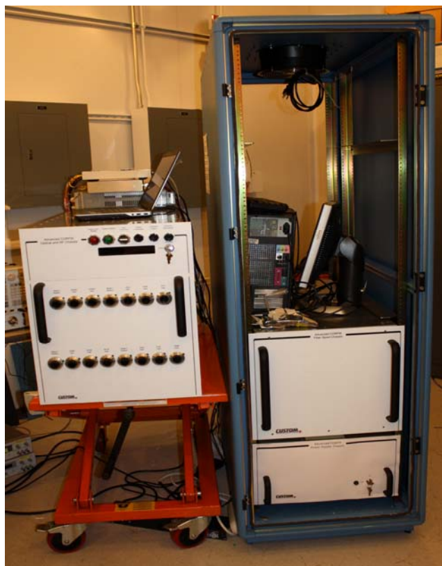
Figure 10. Before Assembly into 19" Rack
